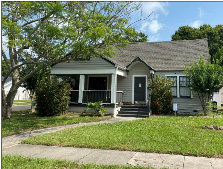
Figure 1: 2020 photograph of subject property by City staff
