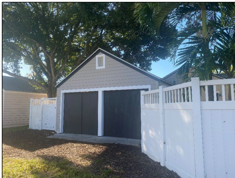
Figure 4: Current photograph of alley elevation of detached garage building
